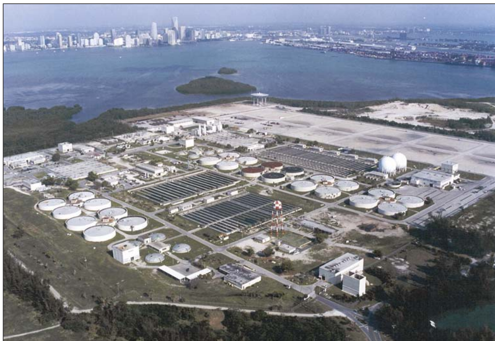
Figure 1. Central District Wastewater Treatment Plant (2012 Existing Conditions Report)
